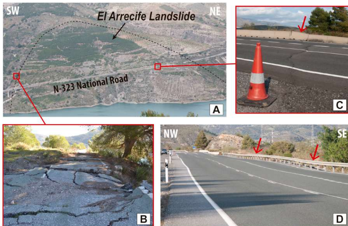
Figure 11. (A) Photograph of the El Arrecife Landslide. (B) Old N-323 National Road in ruins showing opened cracks and partial collapse of the pavement. (C) Bump of the N-323 National Road. (D) Photograph of the N-323 National Road. Notice the ‘waving’ of the crash barrier and the road itself.
