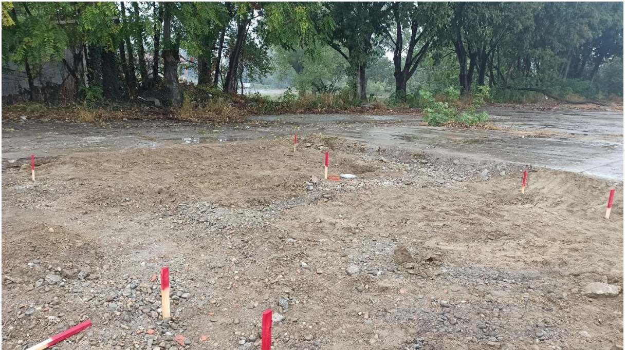
Figure S2. Desealed soil surface after desealing and before to RA addition (October 2023).
